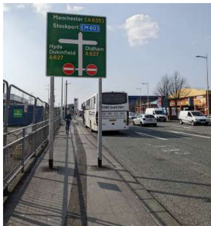
Existing car dominated streets surround Ashton town centre
