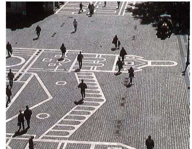
An example of a paving details which define the existing, historic building façades along the street
