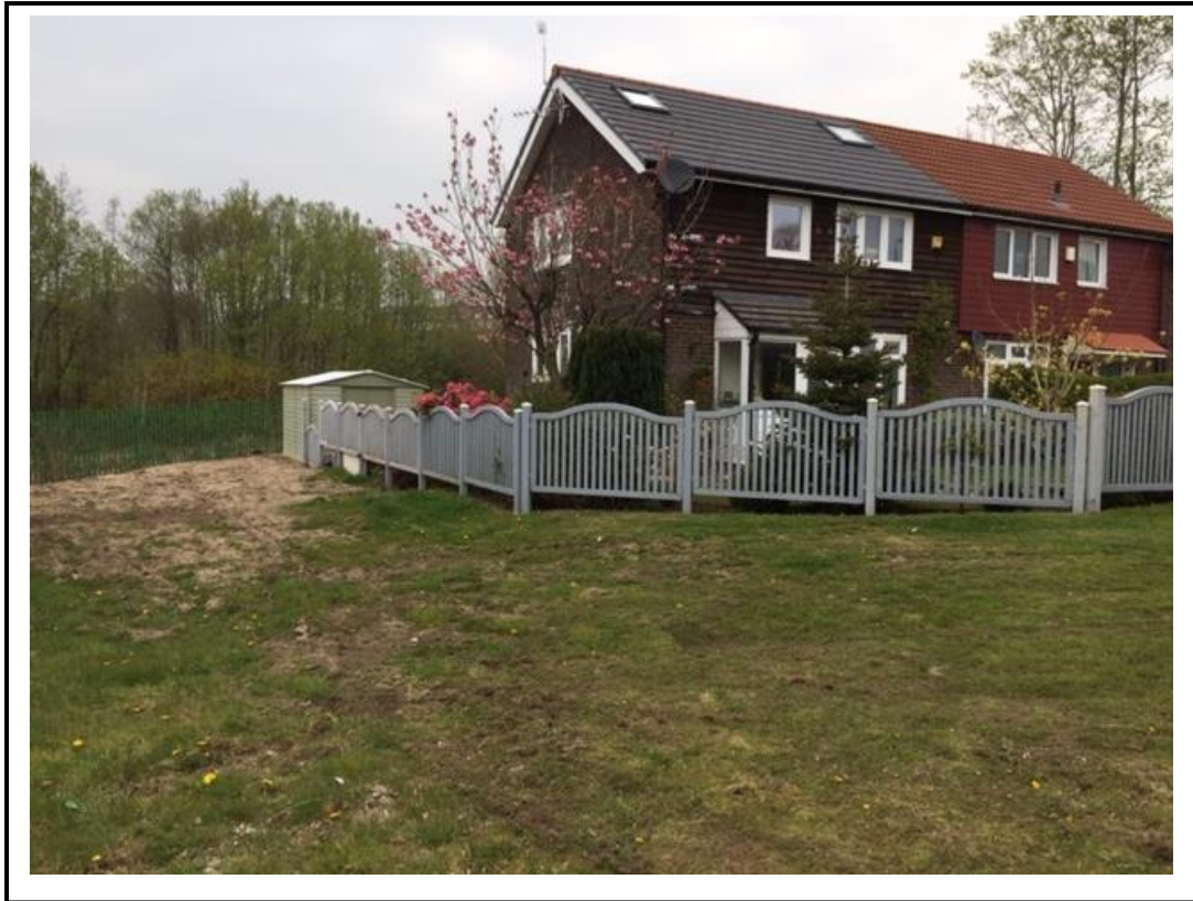
Photo 3 – view of western gable elevation of 14 Milverton Avenue
