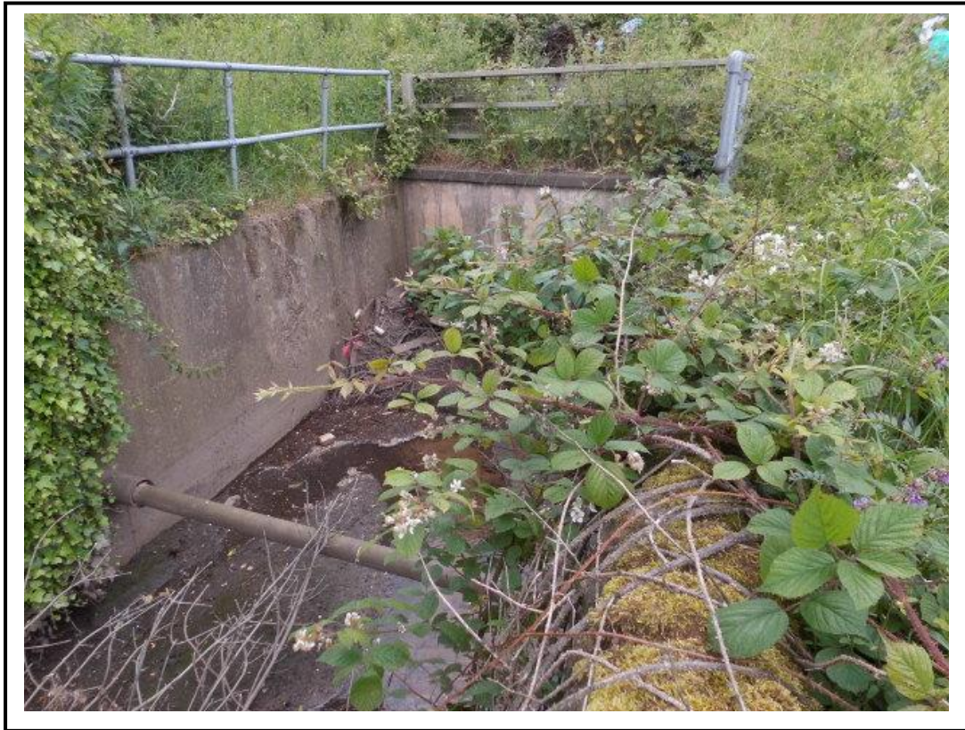
Photo 5: Headwall of Godley Brook before entering Culvert
