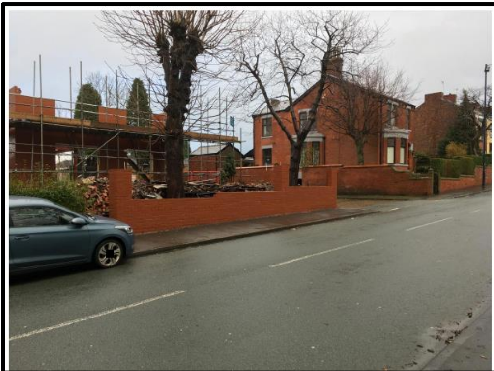
Photo 2 – Site frontage looking east including 213 Two Trees Lane
