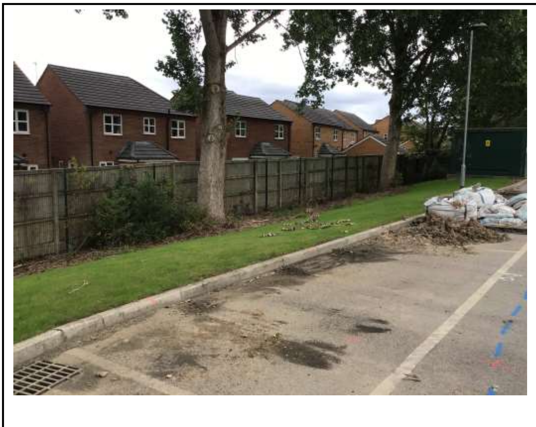
Photo 4 – Part of the western boundary of the school site and properties on Snowdonia Way.
