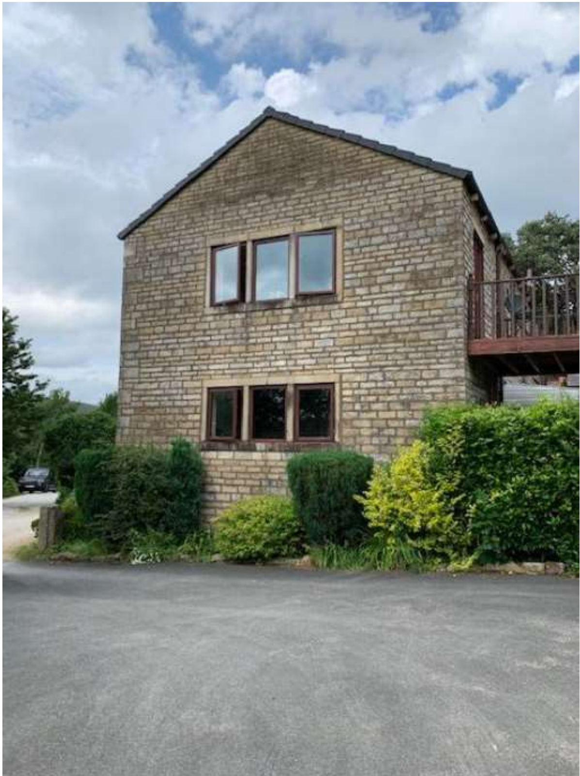
Photograph 3 – Side gable elevation of existing house showing existing two storey side extension and associated projecting balcony
