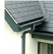
Concrete roof tiles and grey rainwater goods
